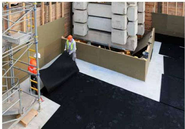
foundation plates, the insulation boards were covered with a standard 2 mm-thick PE film after being installed.
